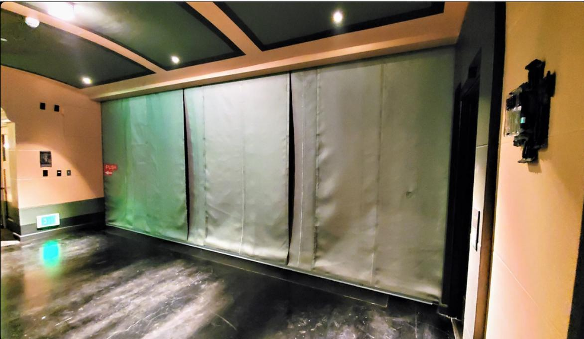
Elevator smoke curtains create a smoke barrier system for buildings that comply with smoke and fire codes. Installing an elevator smoke containment system for smoke and prevention can be done very easily and will eliminate the need for an enclosed elevator lobby.
